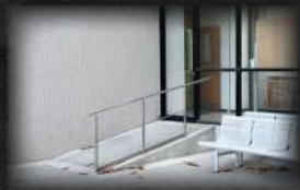
Wheelchair accessible entrance
